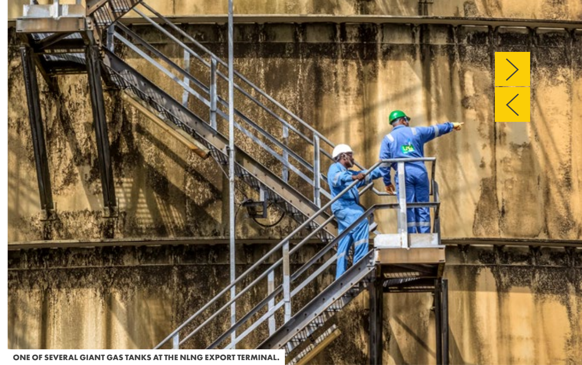
ONE OF SEVERAL GIANT GAS TANKS AT THE NLNG EXPORT TERMINAL.
