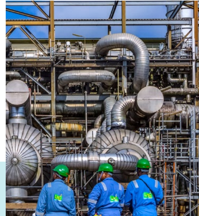
WORKERS AT THE LIQUEFIED NATURAL GAS (LNG) EXPORT TERMINAL AT BONNY ISLAND, NIGERIA WHICH NLNG DECIDED TO EXPAND IN 2020.
